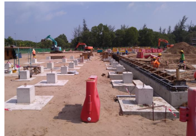
Process and Pipe rack Module Foundation (as of August 2018)
